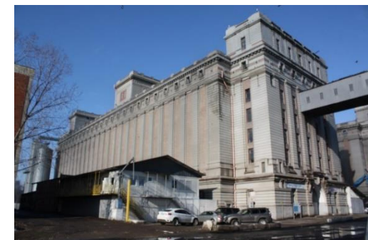
Anghel Saligny Silos, Constanta, Romania
